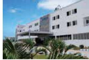
Rudrapur Plant (Green Building)
